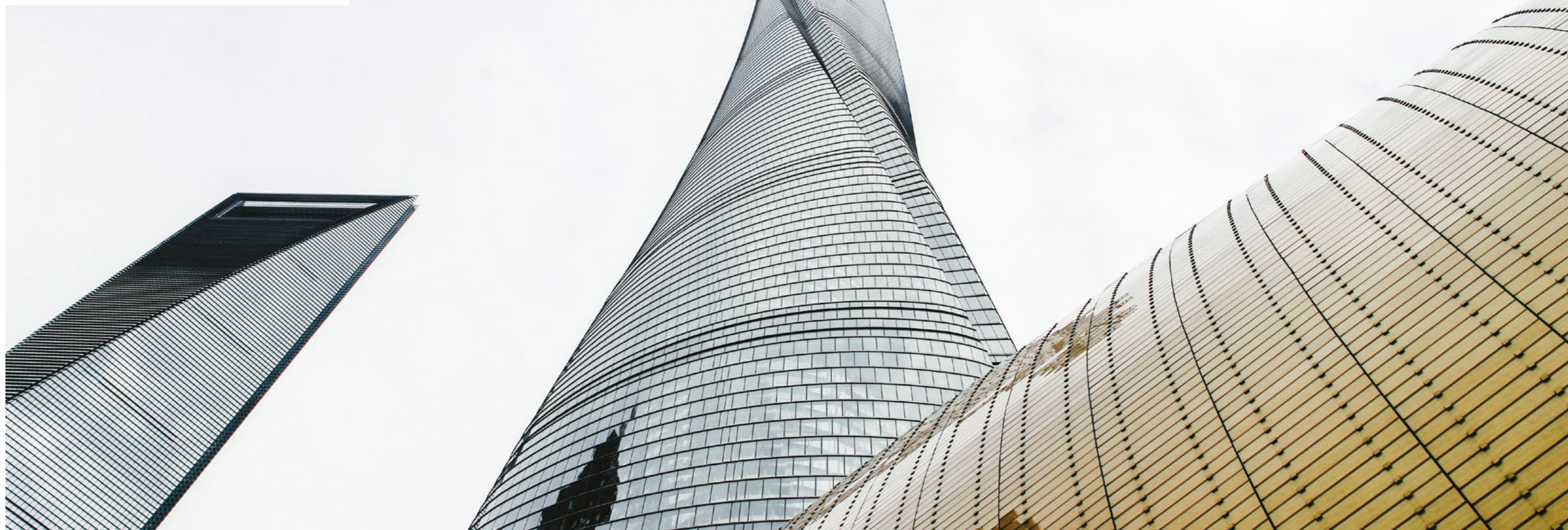
Shanghai Tower, Shanghai
